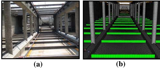
Figure 1: a) Actual image of influent side of the FST, b) Perspective upstream view of CFD model of the FST.
